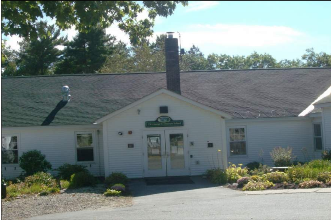
Main entry to Emerson Elementary School.
