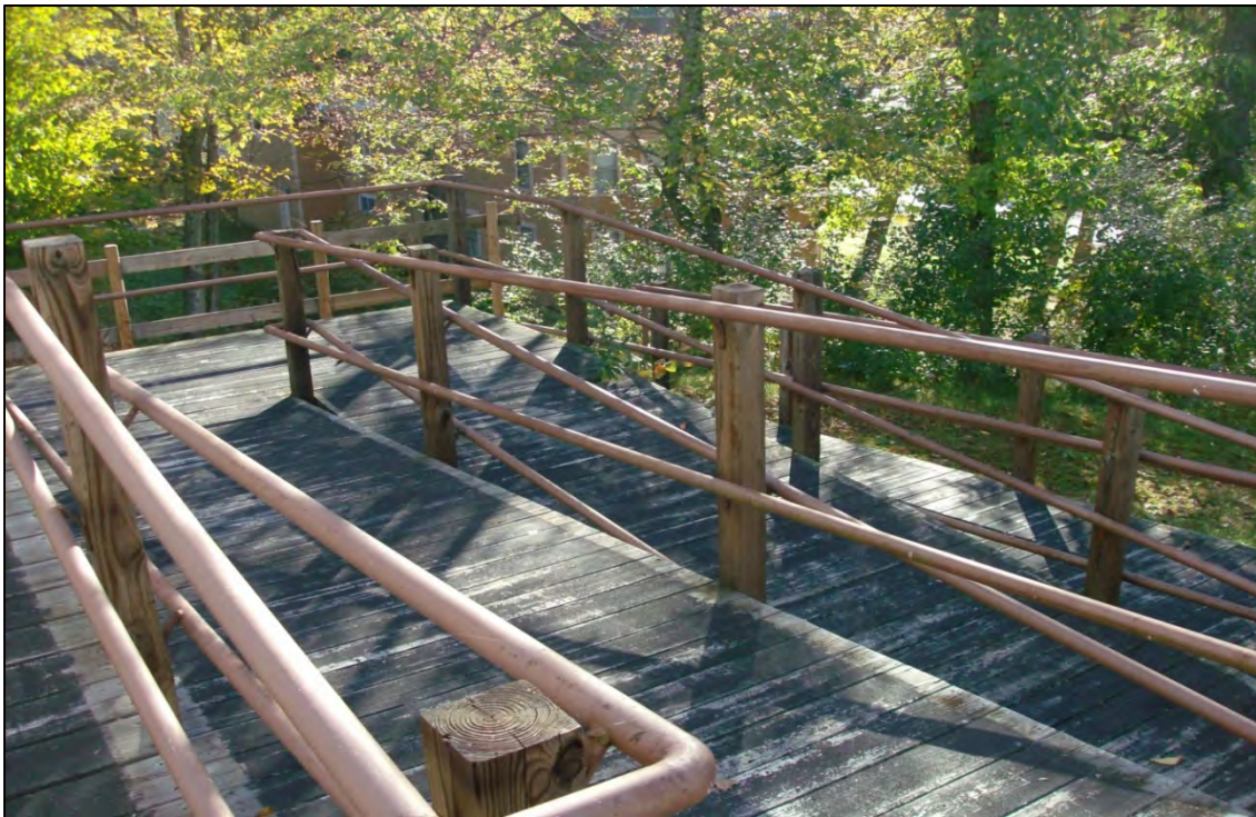
ADA ramp on south side of building with multiple switchbacks.
