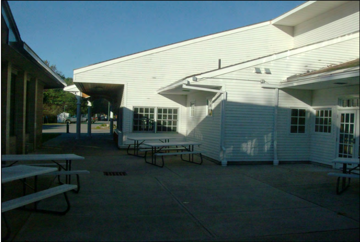
Courtyard area. Note multiple roof slopes directed toward courtyard.
