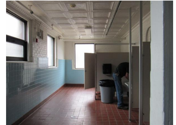
Non-ADA Toilet Facilities
