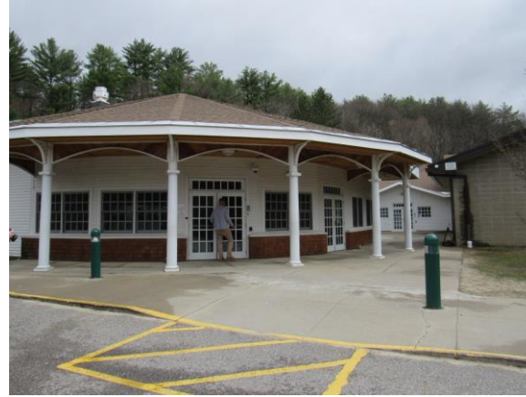
Caf Entrance w/ School Entrance Beyond
