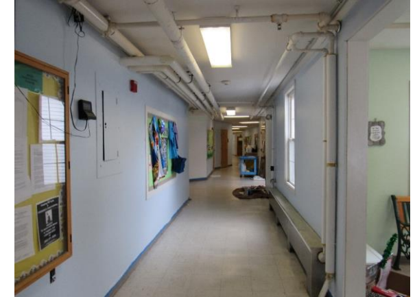
View back to Main Lobby from Principal
