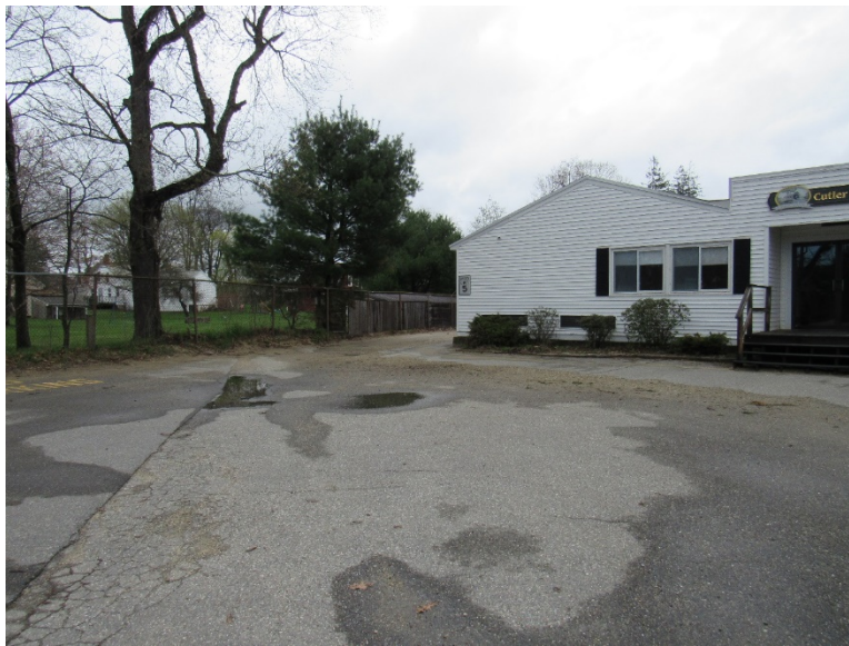
View of narrow alley that busses must pass through.
