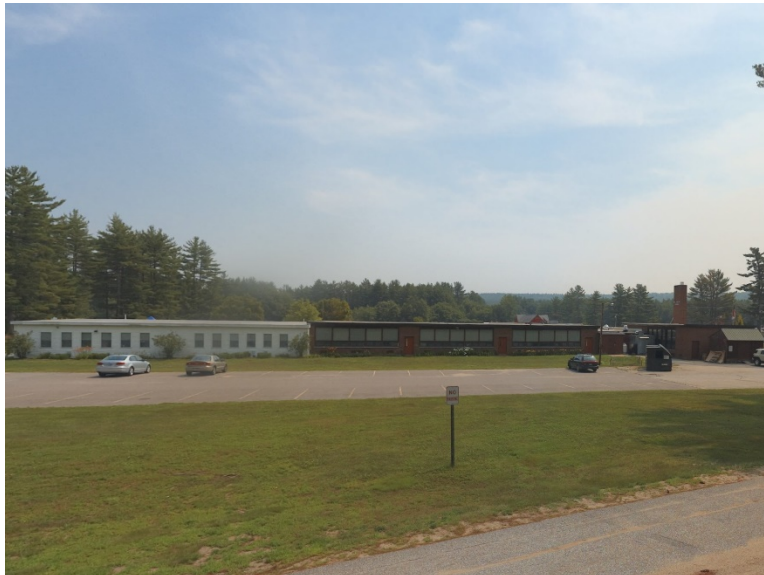
View of side of building.
