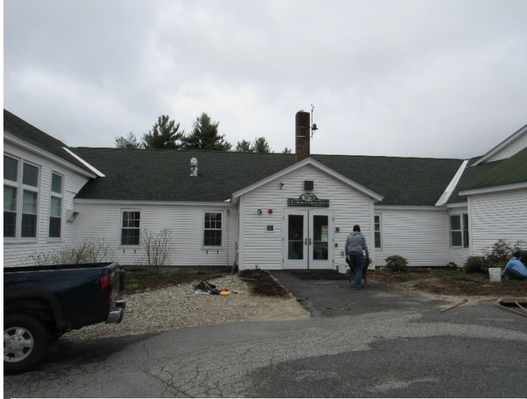
View of main entrance.
