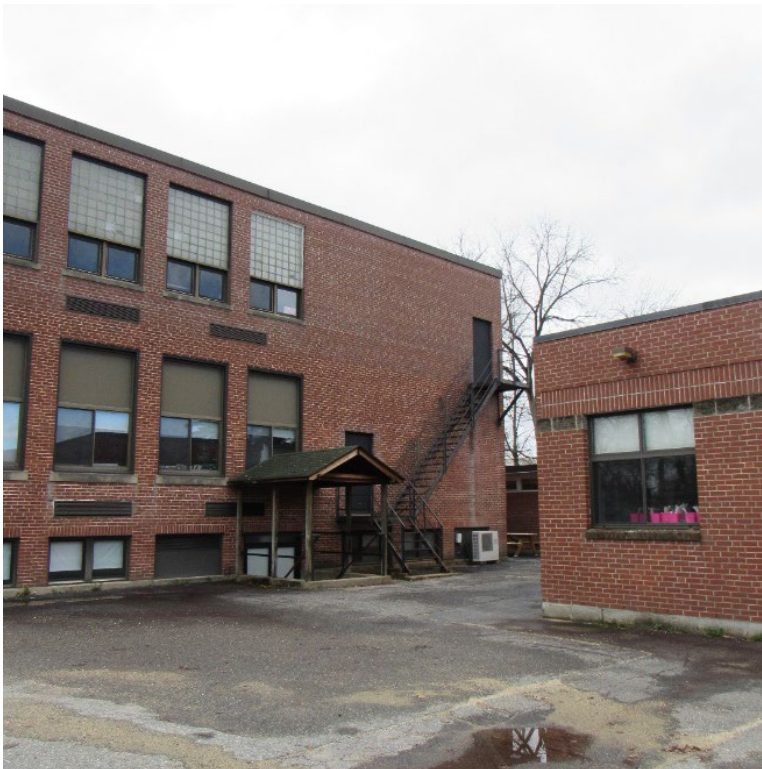
View of the rear of the 3-story structure. Note the fire escape that does not meet code. Note also the courtyard between the building wings that extends to the front lobby.
