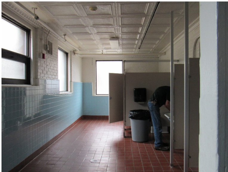
Main toilet facilities.
