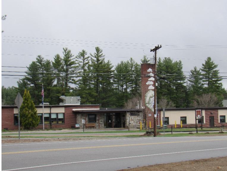
View of front entrance.
