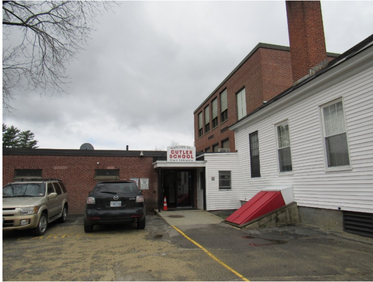
View of main entrance
