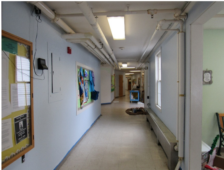
View of main lobby.
