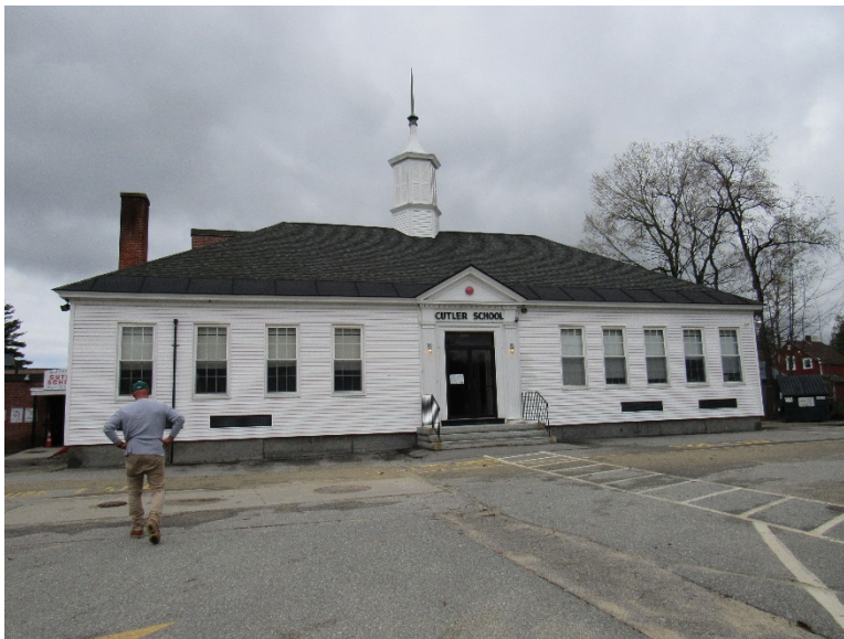
View of historic main entrance now exit only View is from driveway entrance. Note the current front entrance in alley to the left.
