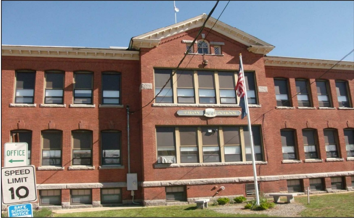
South side of original building. Furnace louver vent behind flagpole.
