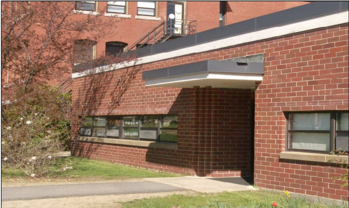
Only accessible entrance on south side of 70's addition.
