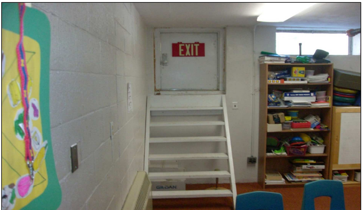
Emergency exit from lower level below the stage.
