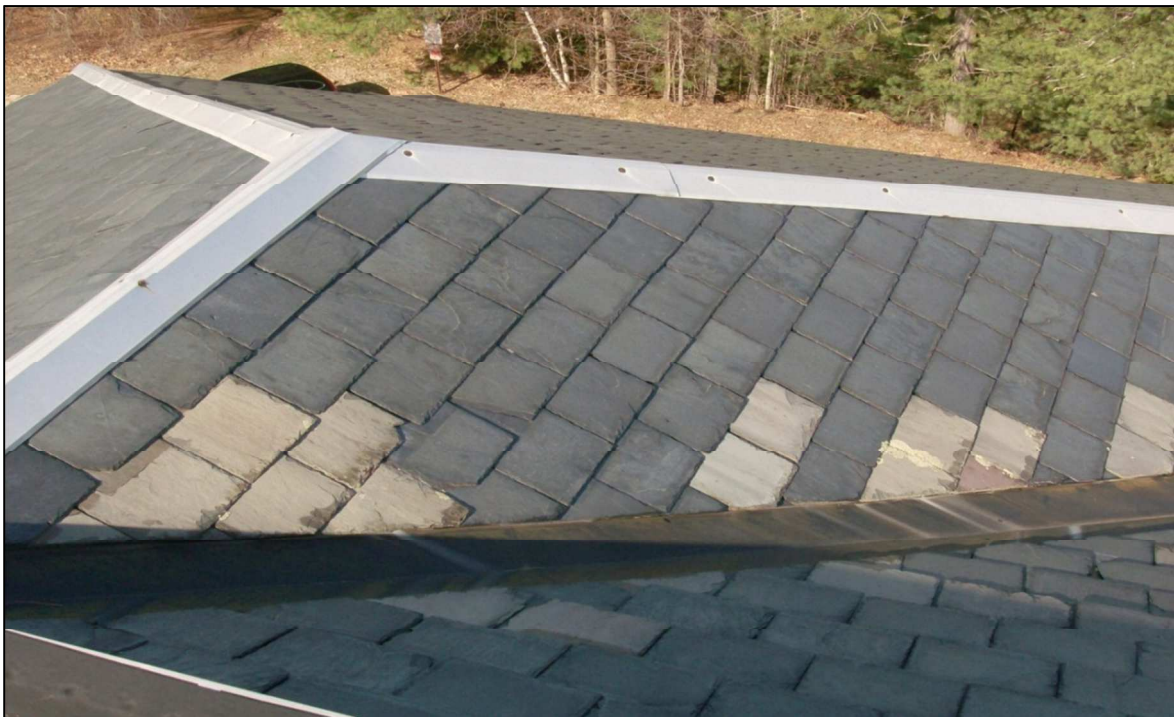
Slat roof over original building. Note replacement slate along the valley.
