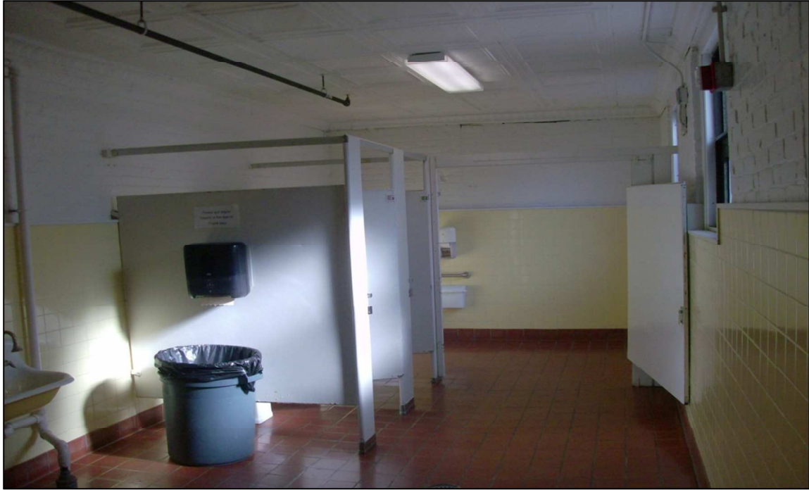
ADA accessible stall in girl's bathroom at lower level.
