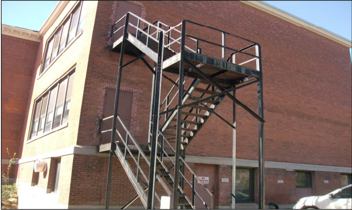
Steel framed stairs on north side of original building.
