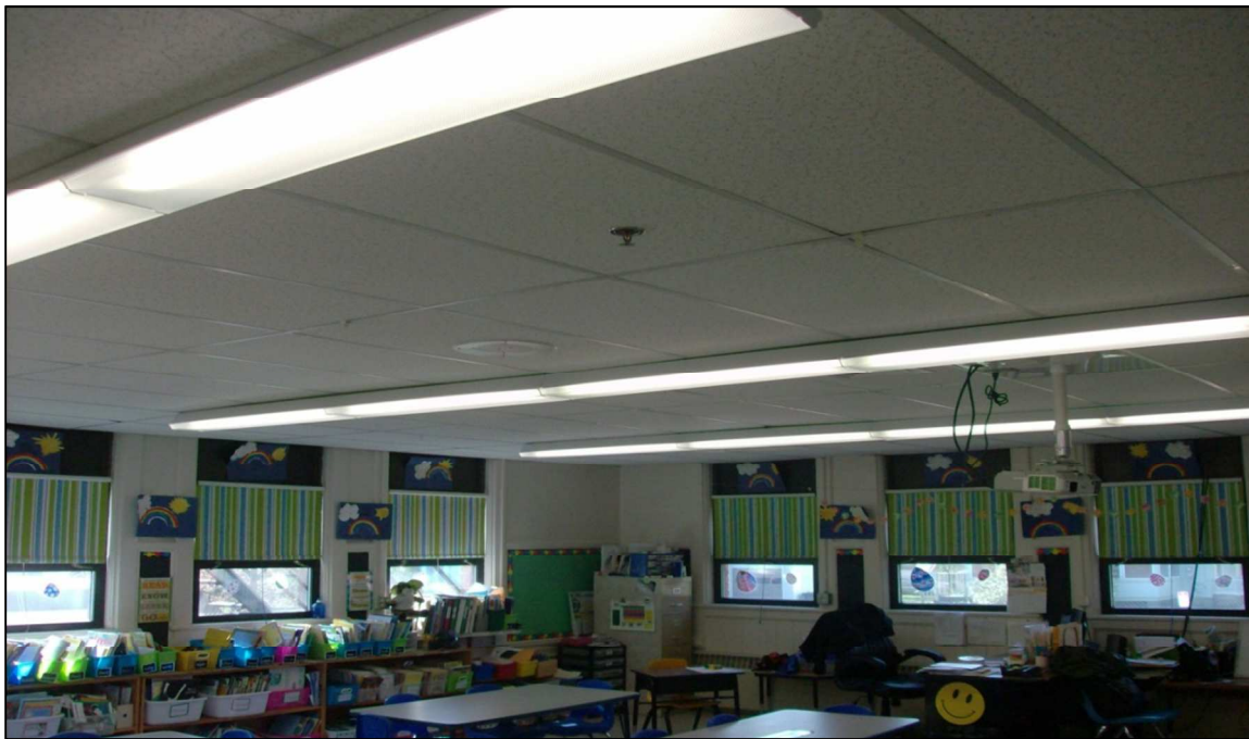
Typical classroom with ACT drop ceiling and outdated lighting.
