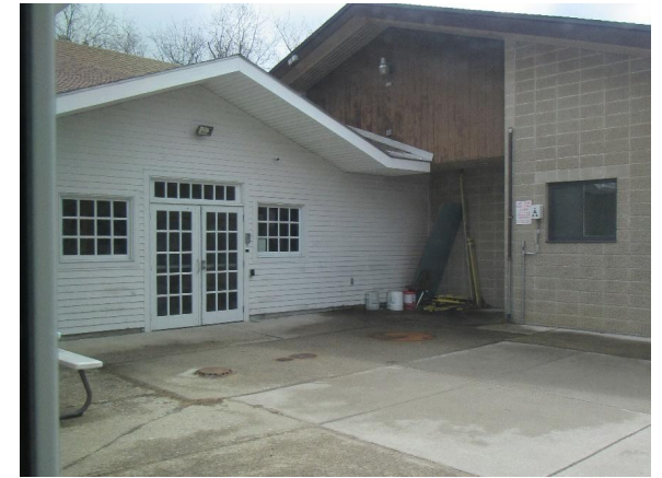
Main Entrance from Courtyard
