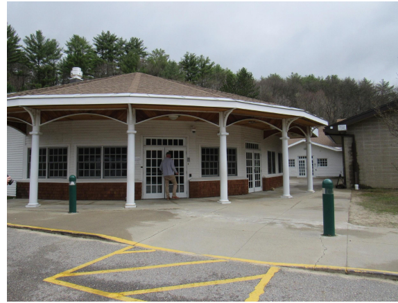
Caf Entrance w/ School Entrance Beyond
